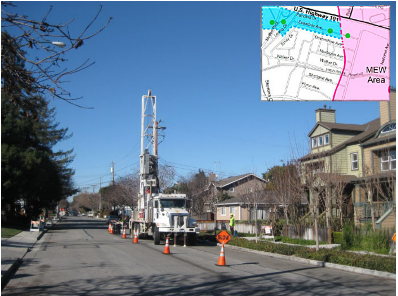
Figure 12. Delineating the plume in the adjacent residential area.
