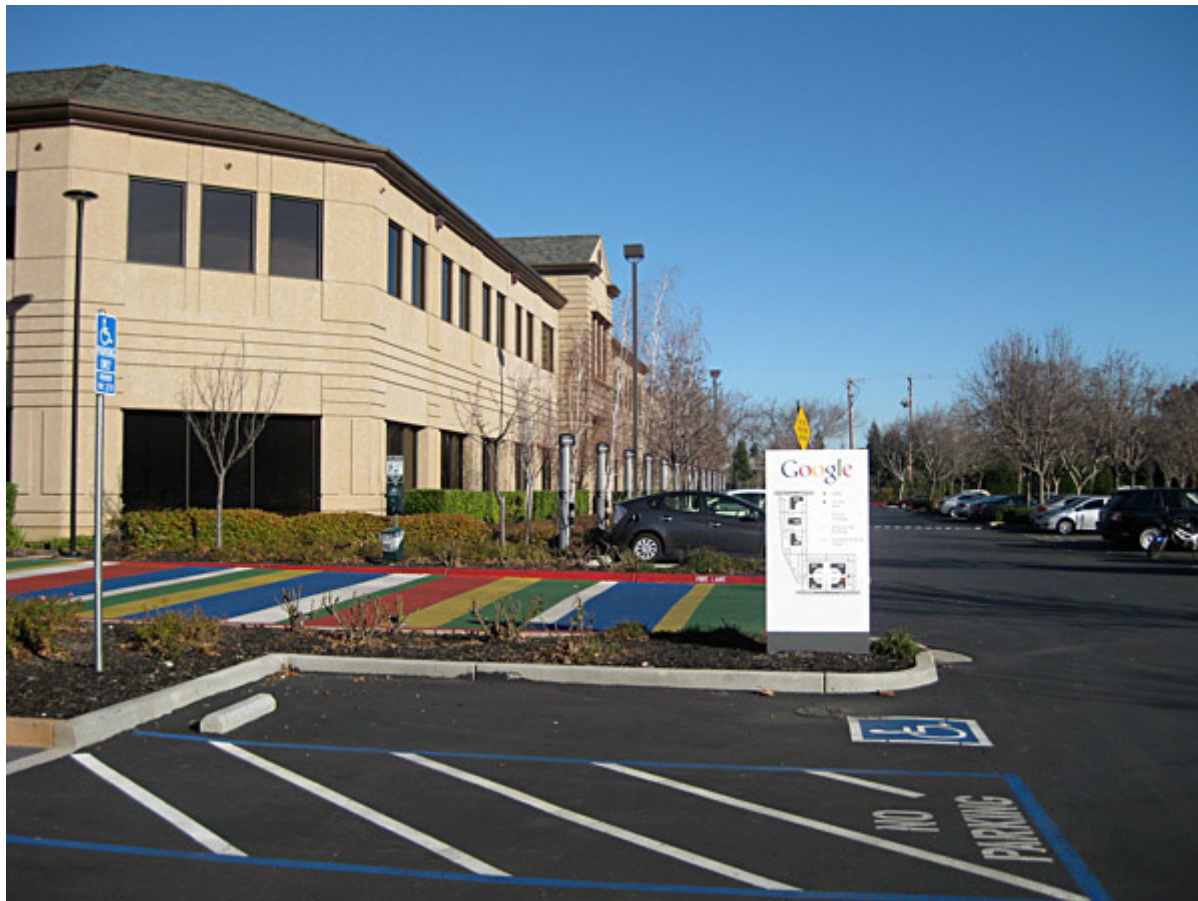
Figure 13. Building where TCE VI is being addressed ( CPEO 2016a ).
