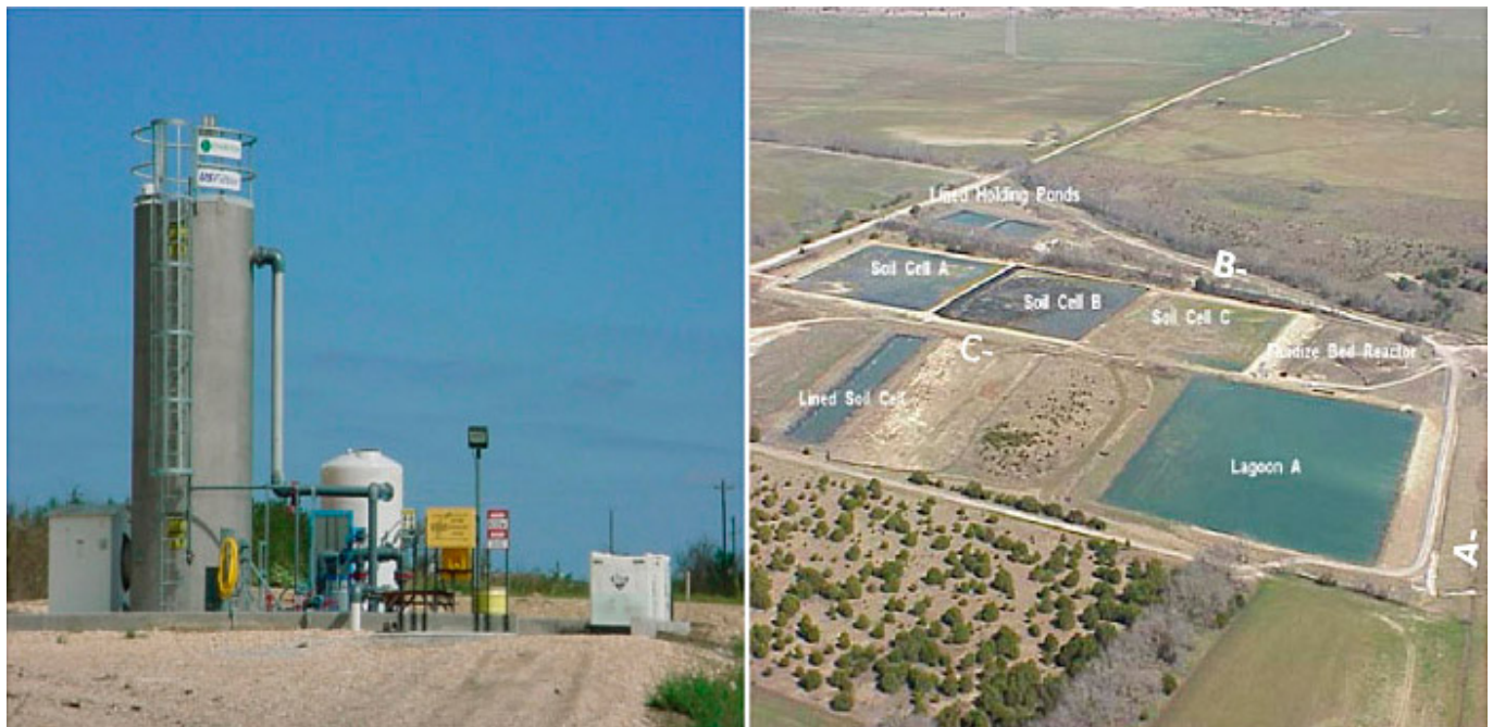
Figure 62. Fluidized bed reactor (FBR) on the left and treatment system components and water management system on the right ( NAVFAC SE, 2016 ).
