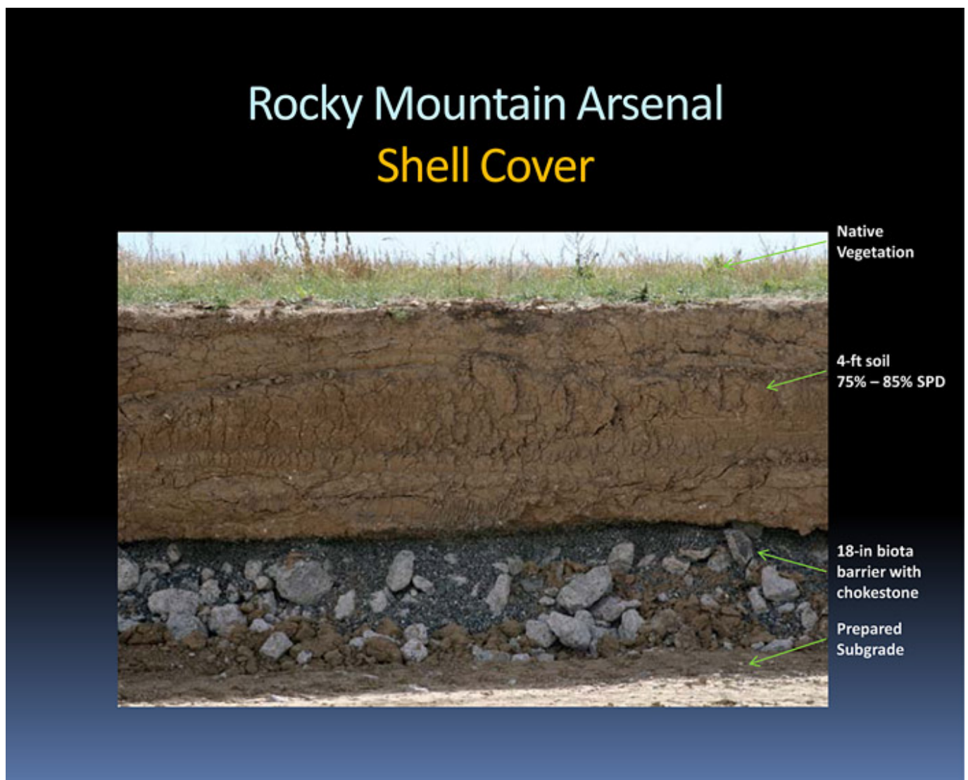
Figure 26. Image of RCRA-equivalent cover cross-section exposed while under construction ( CDPHE 2000 ).
